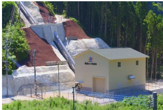
Kamoshishi Hydroelectric Power Plant (Kumamoto Prf., 1,990 kW)
