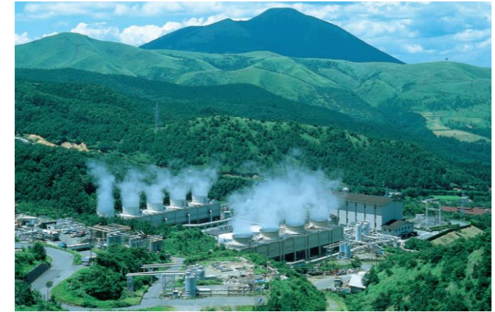
Hatchobaru Geothermal Power Plant (Kagoshima Prf., 110,000 kW)
