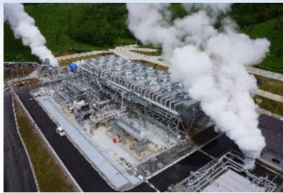
Sugawara Binary Power Plant 5,000kW (operation started in June 2015) ·the first geothermal power generation business in collaboration with local government in Japan
