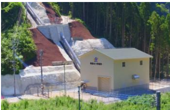
Kamoshishi Hydroelectric Power Plant 1,990kW (operation started in September 2018) ·utilizes the local irrigation and unused fall
