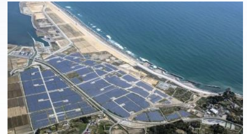
◇Renatosu Soma Solar Park 43,500kW (operation started in June 2017) ·utilizes areas damaged by the great earthquake
