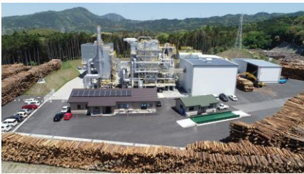
Fukuoka Woody Biomass Power Plant 5,700kW (operation started in May 2020) ·utilizes unused energy of domestic timber as fuel for power generation
