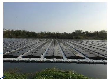
<overseas> Taiwan ◇SuGu I / II Power Plant 5,130kW (operation started in April 2018) ·floating solar power project overseas
