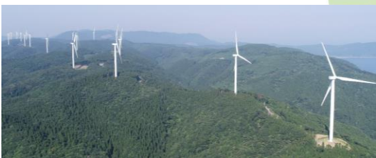
◎Kushima Wind Power Plant 64,800kW (operation started in October 2020) ·23 wind turbine generators
