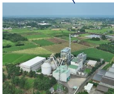
◎Miyazaki Biomass Power Plant 11,350kW (operation started in May 2005) ·uses chicken manure as fuel for power generation
