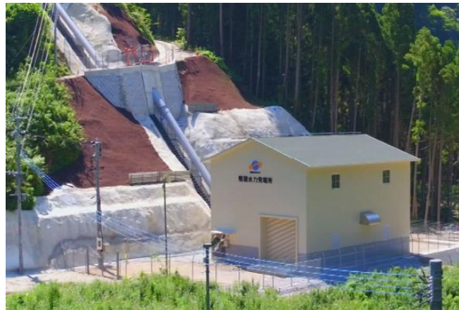
Kamoshishi Hydroelectric Power Plant (Kumamoto Prf., 1,990 kW)
