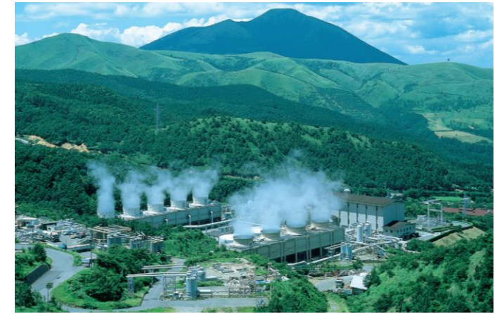
Hatchobaru Geothermal Power Plant (Kagoshima Prf., 110,000 kW)
