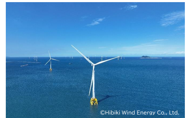
Kitakyushu Hibikinada Offshore Wind Farm (Fukuoka Prf., 220,000kW)
