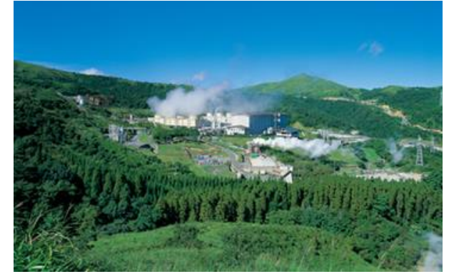
Hatchobaru Geothermal Power Plant (Kagoshima Prf., 110,000 kW)
