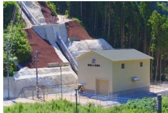
Kamoshishi Hydroelectric Power Plant (Kumamoto Prf., 1,990 kW)
