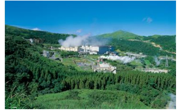
Hatchobaru Geothermal Power Plant (Kagoshima Prf., 110,000 kW)
