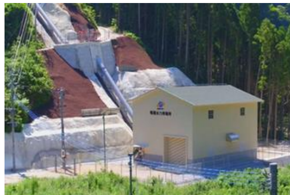
Kamoshishi Hydroelectric Power Plant (Kumamoto Prf., 1,990 kW)
