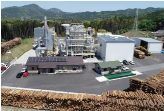
Fukuoka Woody Biomass Power Plant (Fukuoka Prf., 5,700 kW)
